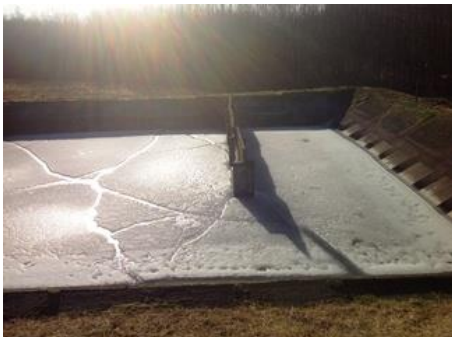
Old biological step reservoir
