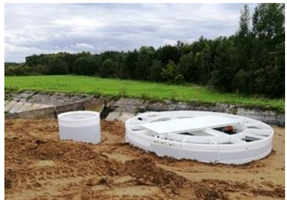
Backfilling of the reactor
