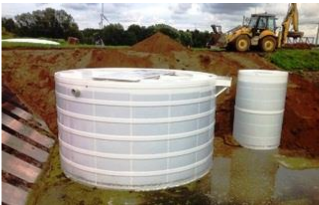
Placing on the foundation
